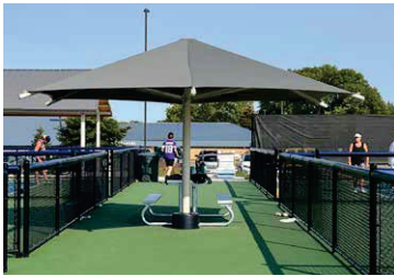
Pickleball Shade Structure
