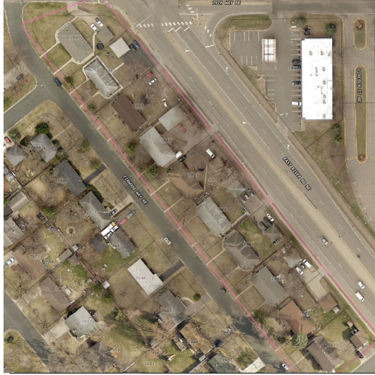
Aerial View of Area
