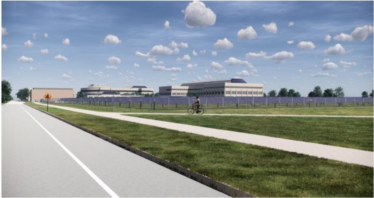
FIGURE 3 – VIEW FROM MEDTRONIC PARKWAY LOOKING EAST
