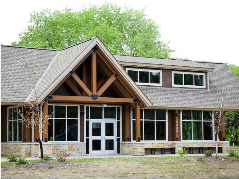
Edina Arden Park Building (interior used as warming house in winter)
