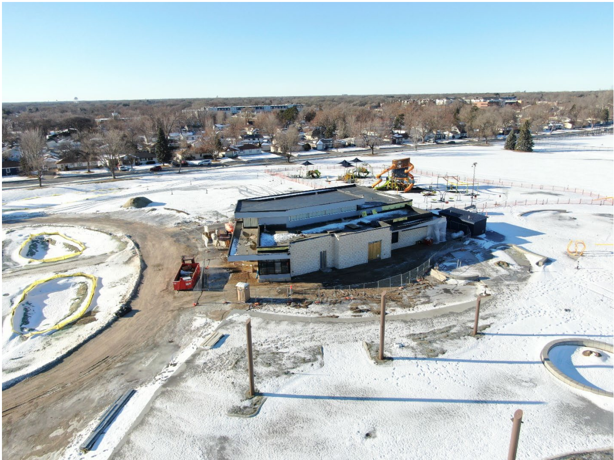
Image of Commons Park Recreation Building construction progress from January 14, 2026
