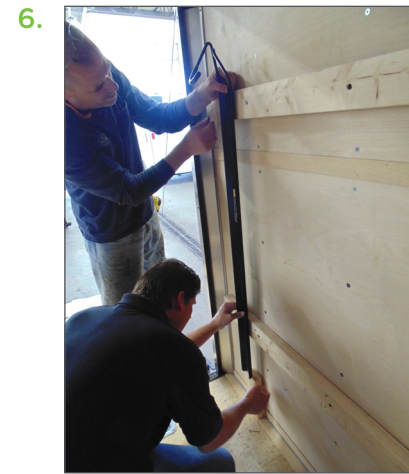
Measuring to ensure the trays are mounted evenly and perpendicular to the floor.
