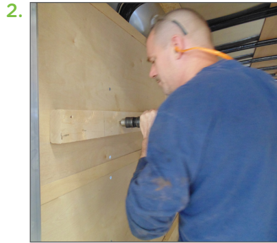
Installation of 2x4" rail to the interior wall.
