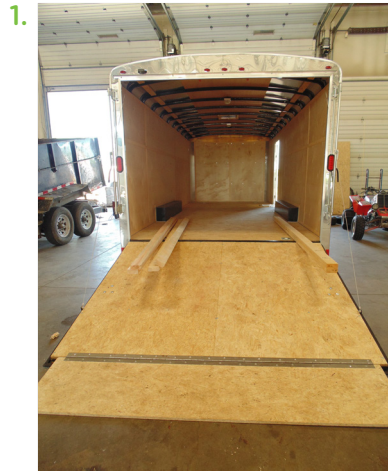
Bare trailer with 2x4" rails to be installed on walls.
