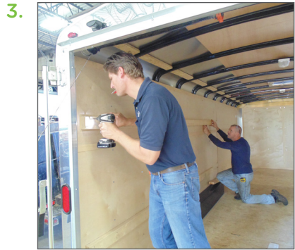
Leveling of the rail.
