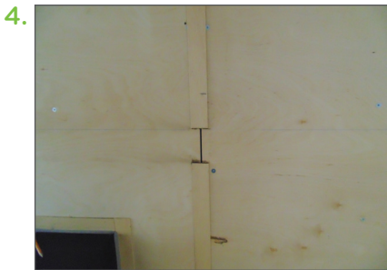
The interior finish may require notching to allow the rails to sit flush against the wall surface.
