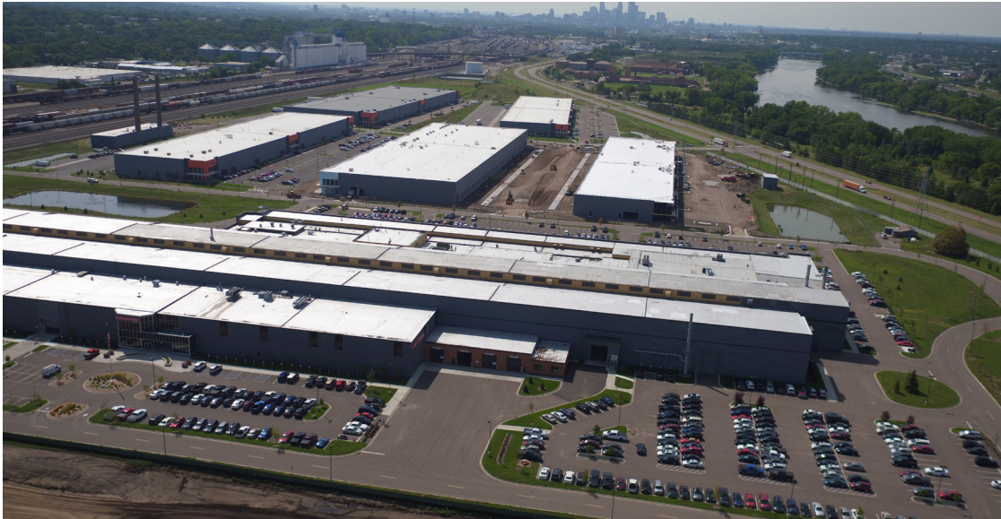
Northern Stacks under construction
