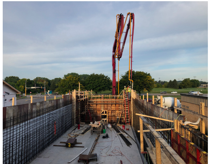
Construction of Locke WTP backwash reclaim basin
