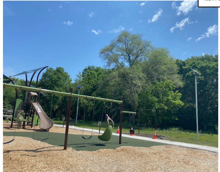
Solar light in the background of Civic Campus Playground
