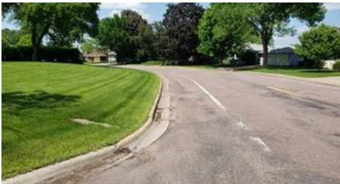
Before and after construction of 7th Street Trail
