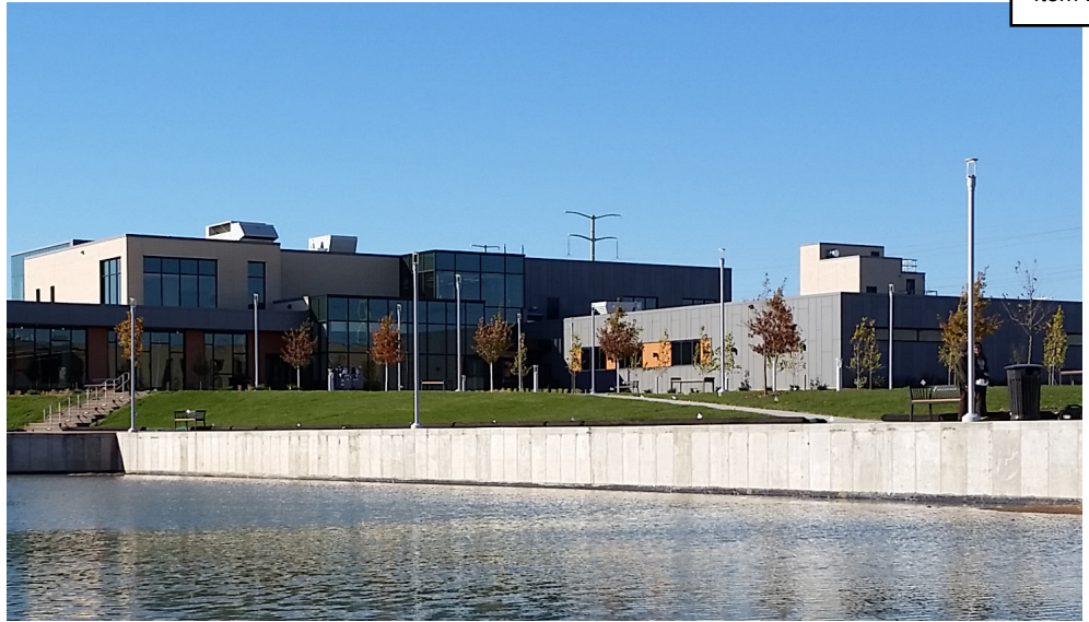
View of Fridley City Hall from Civic Campus Pond
