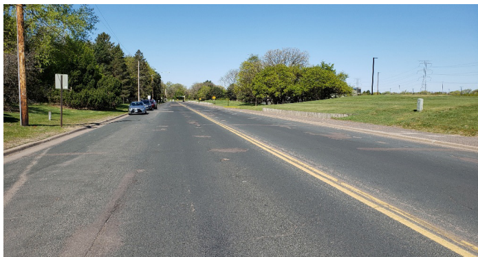
Before and after 69 th Avenue road diet
