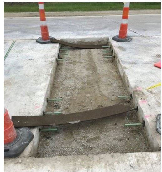
Exhibit 4. Type CD-LV Full-Depth Repair.
