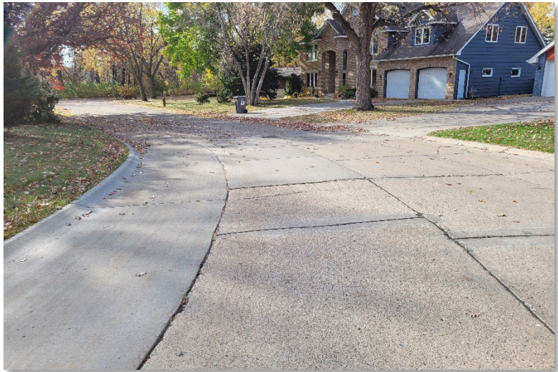
Exhibit 5. Columbia Heights pavement rehabilitation (2024)
