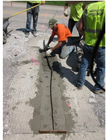
Exhibit 3. Type B3 Crack Repair.
