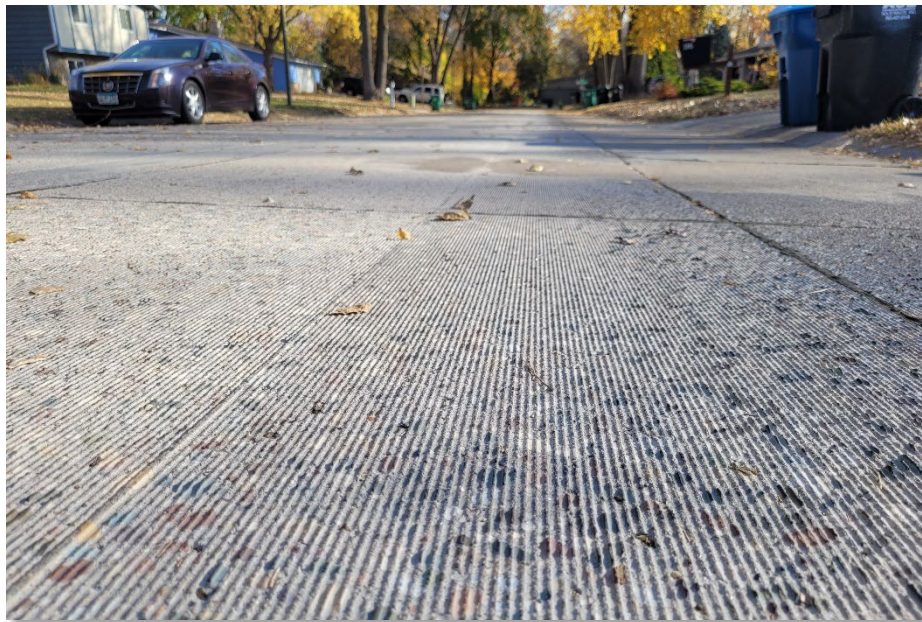
Exhibit 6. Diamond Surface Grinding (New Brighton)
