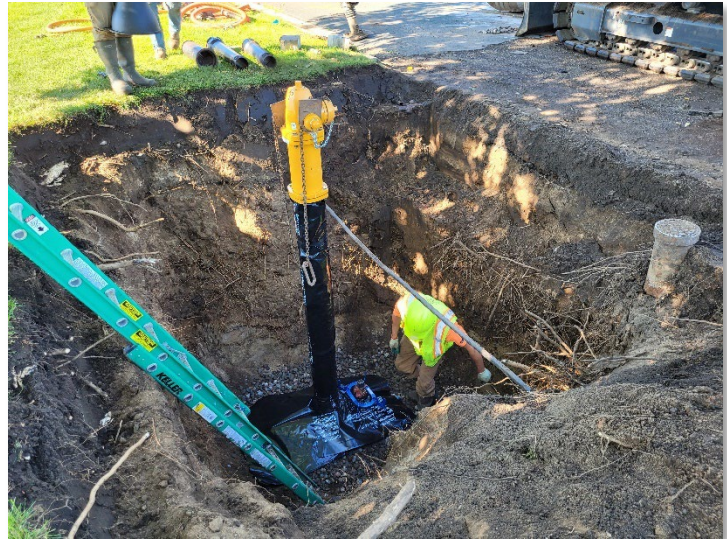
Exhibit 8. Fire hydrant assembly replacement.
