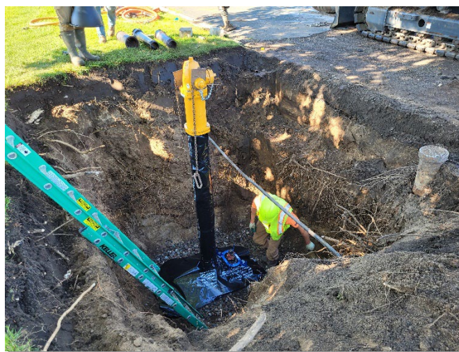
Exhibit 8. Fire hydrant assembly replacement.
