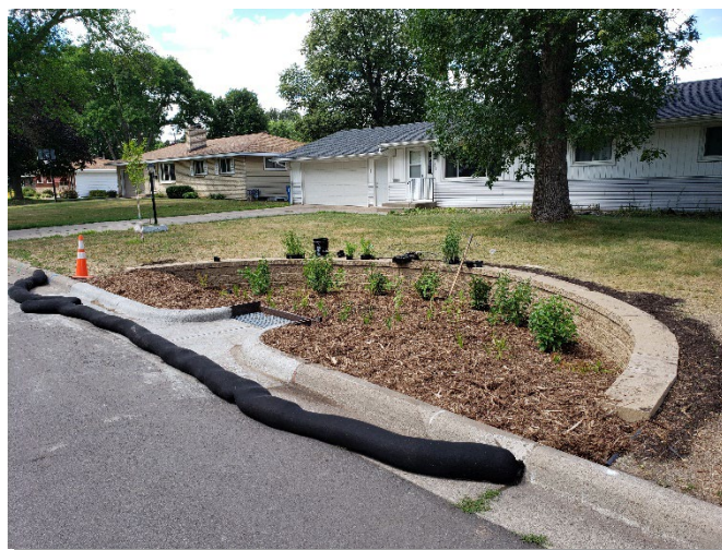
Exhibit 9. Rain garden water quality feature.
