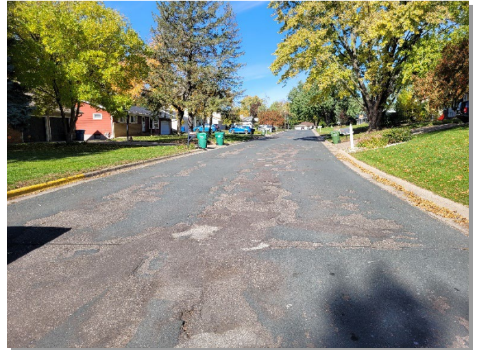
Exhibit 6. Buchanan Street looking south.
