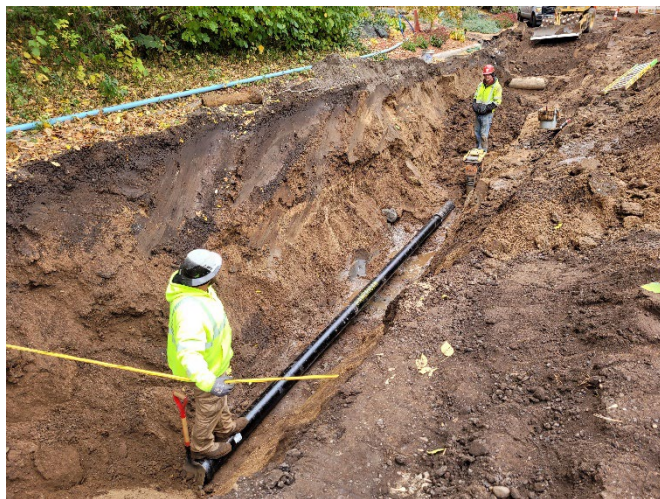
Exhibit 7. Water main replacement.
