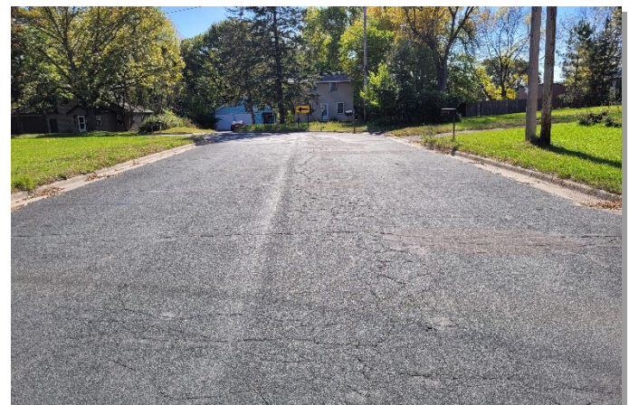
Exhibit 3. Channel Road looking south.
