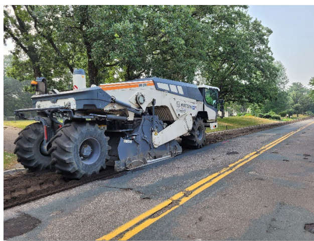
Exhibit 1. Full-depth pavement reclamation.
