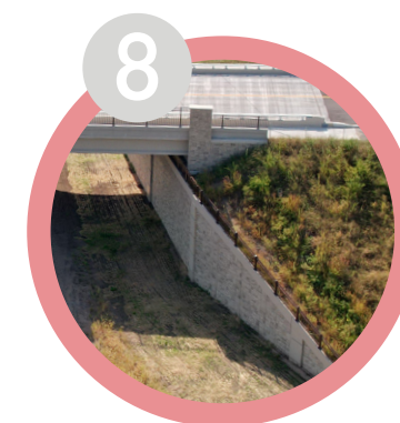
8 Abutment Corner Pylons/Mask
