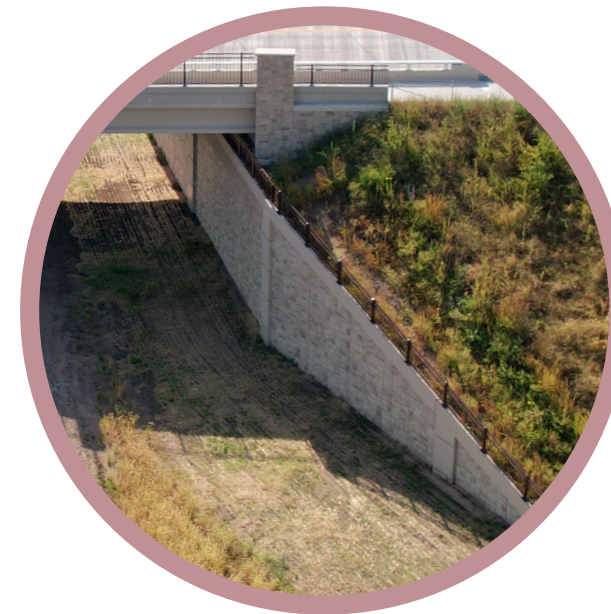
Abutment Corner Pylons/ Mask Walls
