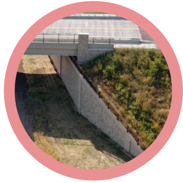
Abutment Corner Pylons/Mask
