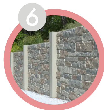
6 Abutment Paint / Texture
