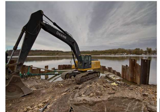
(Public Water Access installation, Mississippi River at Hastings, Dakota County MN)
