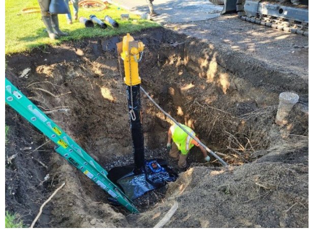
Exhibit 5. Fire Hydrant Assembly Replacement.
