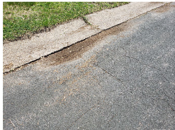
Exhibit 3. Existing Condition at Van Buren Street
