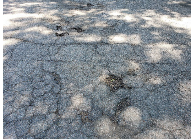
Exhibit 2. Existing Condition at 75 th Avenue
