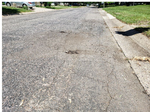
Exhibit 1. Existing Condition at 4 th Street
