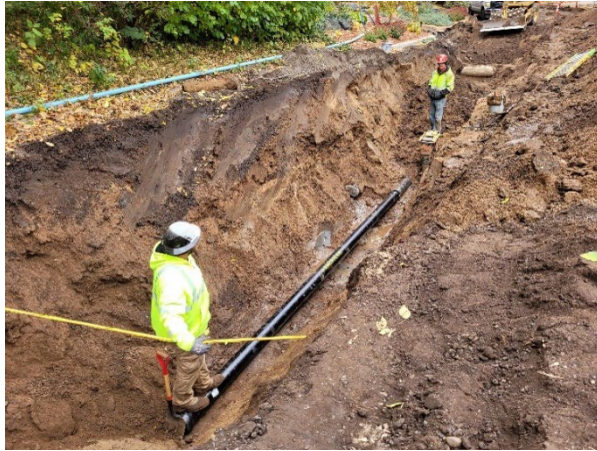
Exhibit 4. Water Main Replacement.
