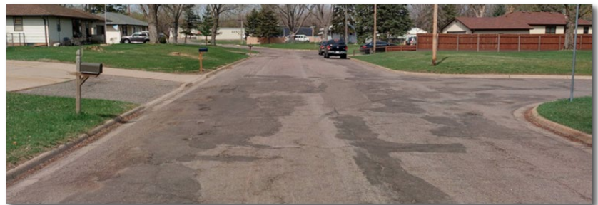
Exhibit 3. 63 rd Avenue looking west.
