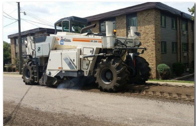
Exhibit 1. Full-depth pavement reclamation.
