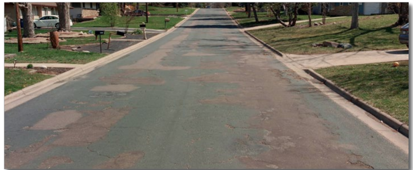
Exhibit 4. Skywood Lane looking east.
