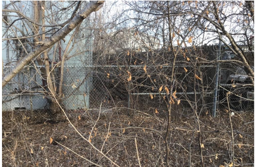
Figure 1: The current chain link fence, viewed from BNSF right-of-way on February 1, 2024. The fence has been cut and repaired (center of the image). Easily climbable vegetation grows through the fence. The fence is shorter than the adjacent southern property's fencing.
