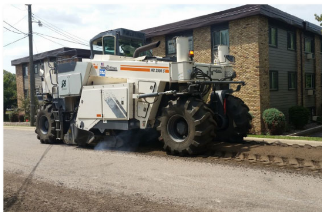
Exhibit 1. Full-depth pavement reclamation.
