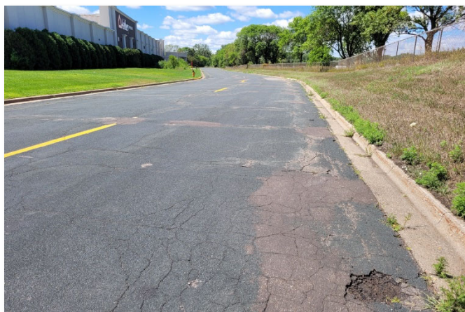
Exhibit 3. East River Rd Service Drive looking south.
