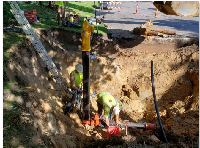
Exhibit 6. Fire hydrant assembly replacement.
