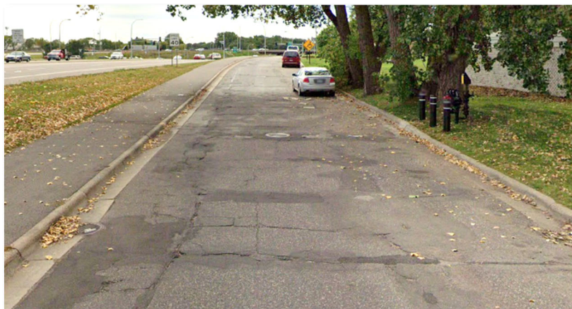
Exhibit 4. East River Rd E Service Drive looking south.
