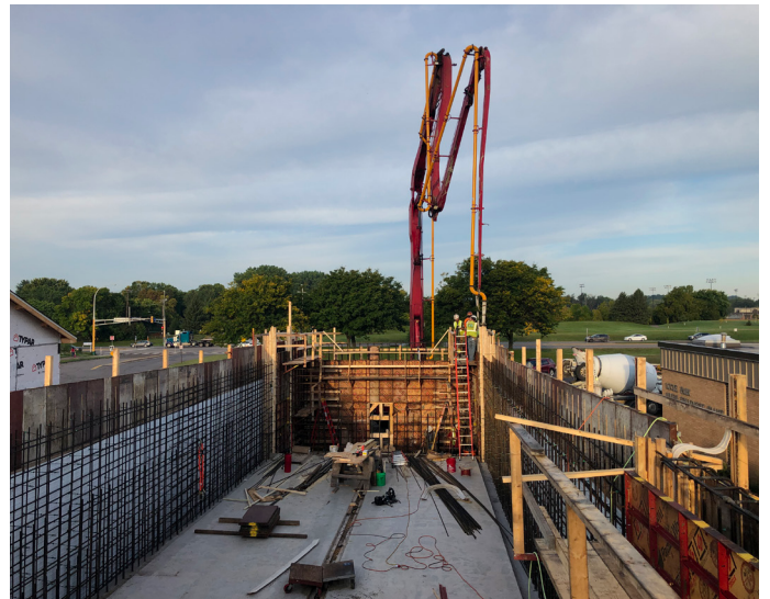
Construction of Locke WTP backwash reclaim basin
