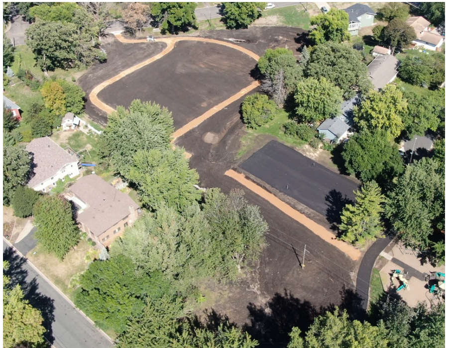
Aerial view of Craig Park project during construction
