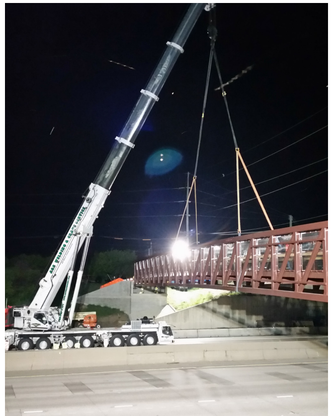
Installation of Main Street Bridge
