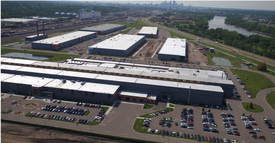
Northern Stacks under construction
