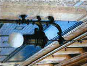
Artisans unknown, Hamm Building, Saint Paul, MN, Tolitz, King, Day Architects
