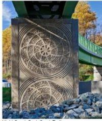
Vicki Scuri, Rock Creek Trail, Pedestrian Bridge, Photo © Roger Foley
