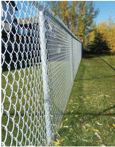
Galvanized Chainlink Fencing
